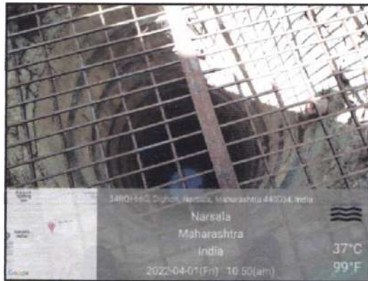
Wells situated in College Premises 2
